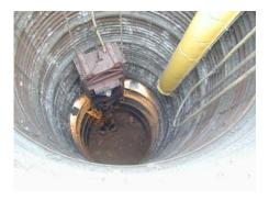
The analyses indicated that without grouting, inflows to the shaft of hundreds of gallons per minute might be anticipated. With an average grouting program, these flows could be reduced to tens of gallons per minute. An intensive grouting program was subsequently carried out that reduced inflows to less than 25 gallons per minute.
