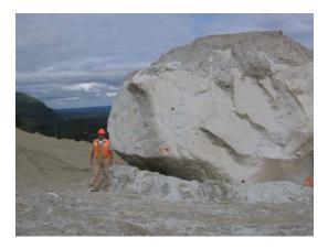
The boulder was successfully split into pieces that could be handled by the on site equipment without any fly rock.
