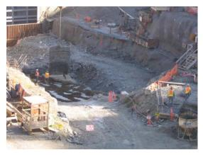
The photograph below shows a sidewall blast that was successfully drilled, loaded, matted, and shot just above the waterline.
