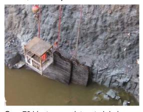
Over 70 blasts were detonated during Phase I excavation with all recorded vibrations below 16 in/sec and no observed structure damage.
