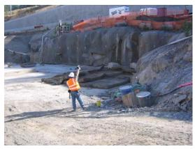
This photograph shows an initial sinking shot located about 100-ft from the intake tower and bridge structure.
