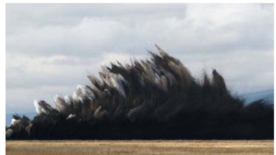
Left: Regional map showing restoration area and four breach sections. Above: One of the half-mile sections of levee is "unzipped" in a matter of a few seconds.
