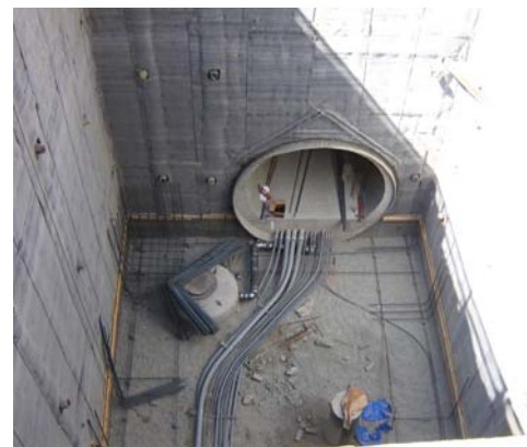
The photograph above shows the lined completed tunnel with utility conduits embedded in the slab.
