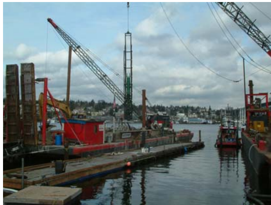
This photograph shows the crane mounted vibratory hammer installing a dock piling.
