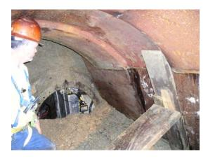
The large diameter pipe reached the MTBM within an inch of line and grade as shown in the photograph above.
