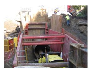
**SubTerra** personnel observed installation of the recovery tunnel and the tunnel face on encountering the TBM.
