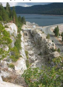
Construction is expected to be accomplished using drill-and-blast methods with smooth-wall blasting of the final cut slopes. Ground support requirements are likely to be minimal but
