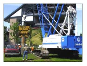
Construction specifications for pile driving required that Peak Particle Velocities (PPV's) during driving be kept below 0.25 in/sec for 72-hr or younger concrete, and 0.5 in/sec for older and pre-existing concrete.
