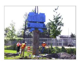
Vibration monitors were situated at various distances from the pile driving operations, in order to identify a relationship between PPV and distance. The relationship thus obtained allowed prediction of pile driving effects on preexisting structures, and recommendations for minimizing these effects.
