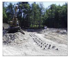
vegetation had been stripped from the development site and footing excavations had been completed for most of the planned structures. Four existing offsite structures were sufficiently close to the planned
